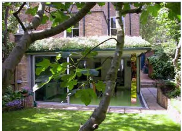
*Figure 16: An extensive green roof Courtesy of Sall, Cullinan and Buck Architects Ltd.*
