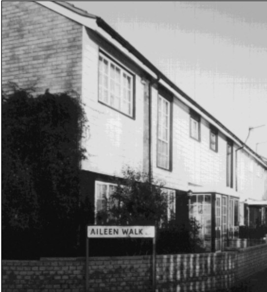
Careful matching of materials and details makes the extension indistinguishable from the original house
