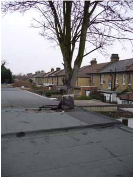
Buildings constructed too close to an existing tree
