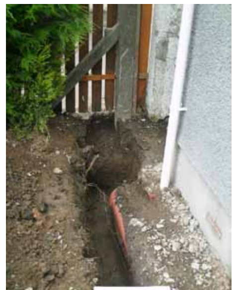
Drains frequently run along the side or back of houses which can sometimes affect the extent of an extension
